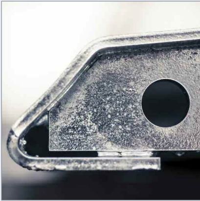
Air lock prevention. The photo shows how stopping short the end plate prevents an air lock.
