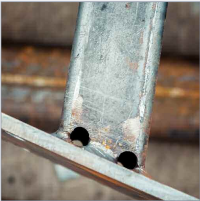
External venting in hollow section frames. The photo shows a RHS fabrication. The hole size is adequate.
